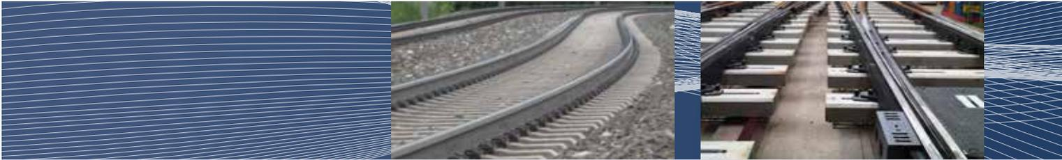
**Modern track bed structures** require elastic components to minimise the forces produced by the weight and speed of trains and damage on wheel and rail running surfaces as trains pass over them.
